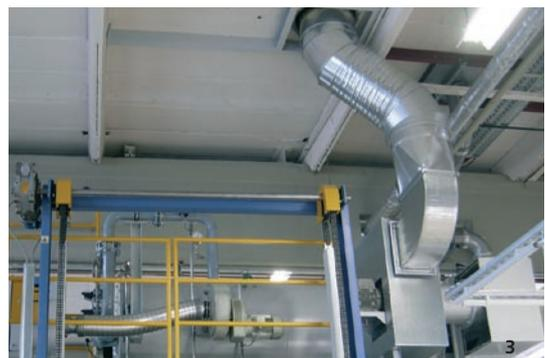
(1) Gas fired thermal afterburner with suction fan and switchgear
